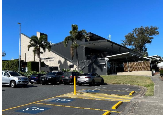
Picture 2 – Victoria Park function centre Source: Urbis Pty Ltd
