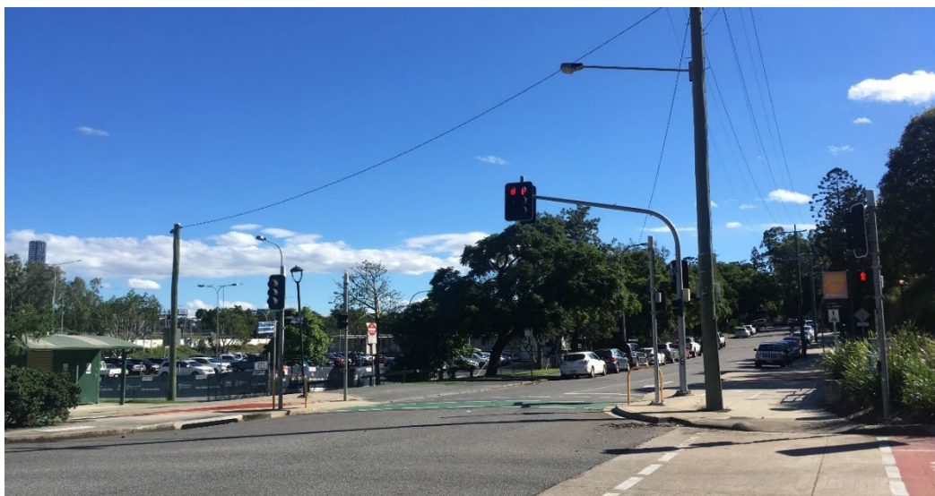
Picture 27 Looking south to where the bridge will cross Gilchrist Avenue.
