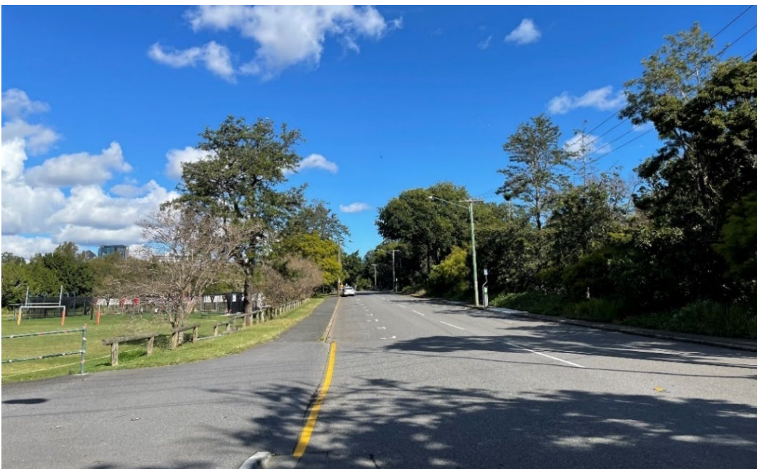
Picture 21 Looking south towards where Gilchrist Avenue will terminate.
